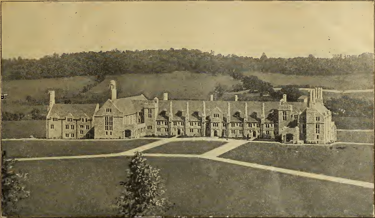
Grounds of the new Masonic Homes, Elizabethtown, Pa. (showing Grand Lodge Hall), sown exclusively with Michell's Grass Seeds. The Committee having in charge the installation of the buildings and the arrangement of the grounds, after exhaustive inquiry and reports on purity and germination tests of Grass Seeds, awarded us the entire contract for supplying Grass Seeds to sow their immense tract of lawn.
